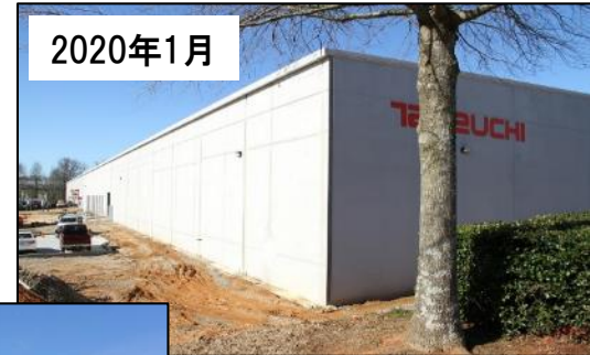
Takeuchi US 倉庫増築 (約5.4億円)
