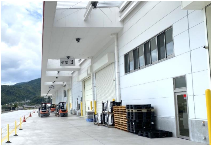
Receiving area at Aoki Factory
